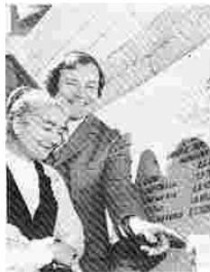
Vida Horn and Ivan Trayling inspecting the library foundation stone, August 1972 Photo: St Kilda Today , No 3, Aug 1972
