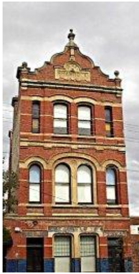
Former Shannon and Shamrock Hotel, 2003
