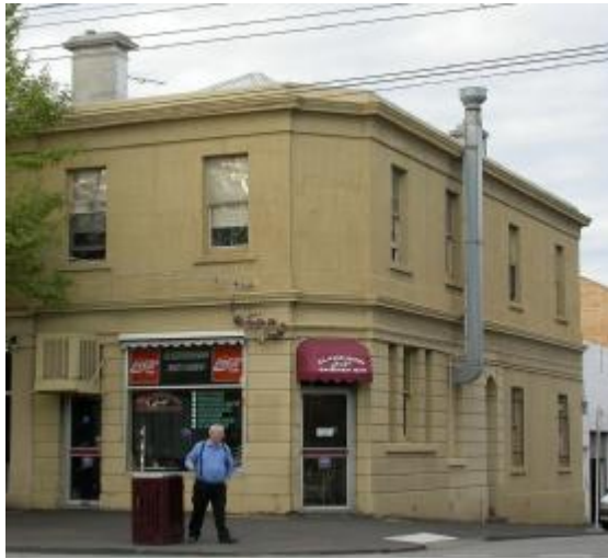
Site of former Criterion Hotel, 2004
