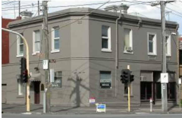
Site of the former Crescent Hotel, 2004
