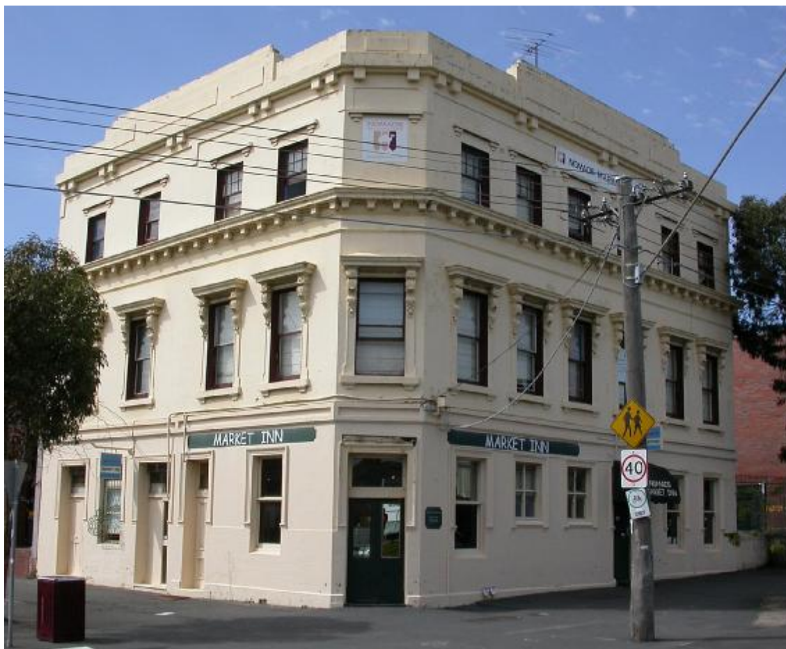
Market Inn, the former Council Club Hotel, 2004
