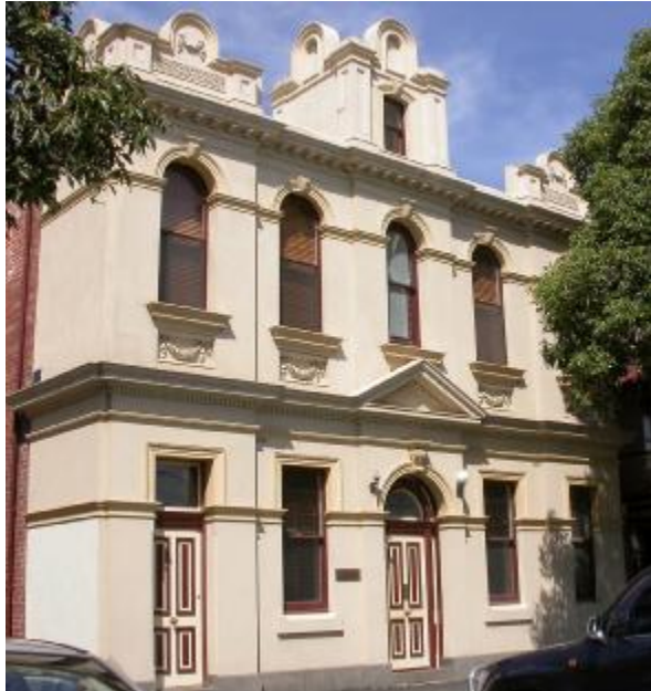
Site of the former Caledonian Hotel, 2004
