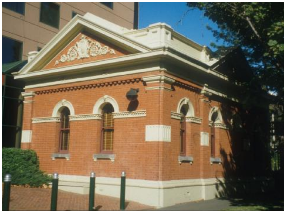
Former Gas Valve House, 2002
